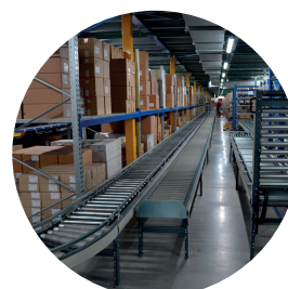
Warehouse complex of “BaDM” corporation, Dnipro
